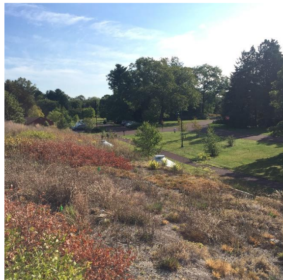
Figure 12. Intensive Green Roof
