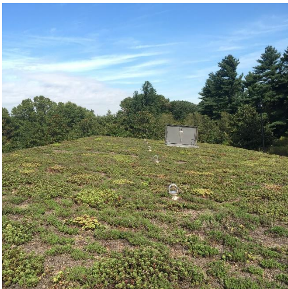
Figure 11. Extensive Green Roof
