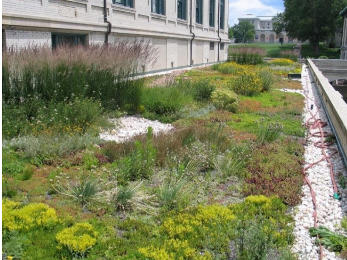
Figure 6. Shallow Layer of Gravel along the Roof Perimeter
