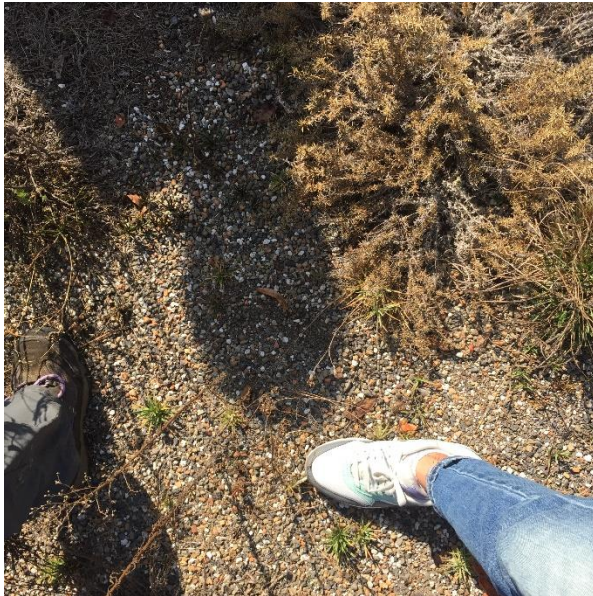
Figure 7. Green Roof Growing Medium
